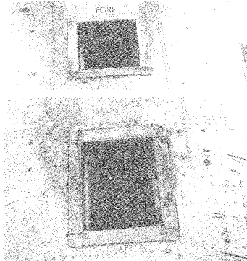
Figure 19. Two static vents 22.9 by 30.5 cm (9 by 12 in.) mounted on the top of the B-25 Mitchell tank.
