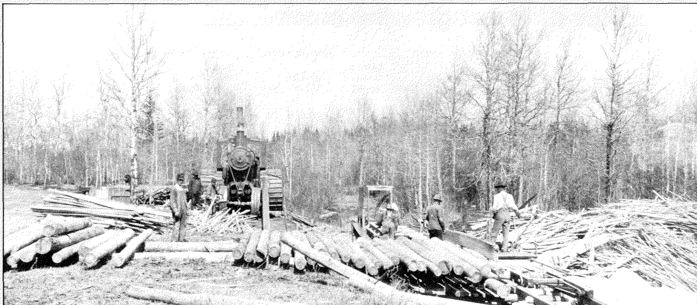
Mobile steam-powered sawmill, 1910
