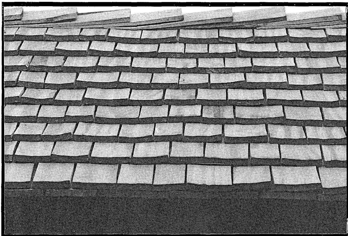
Figure 37. Black Gum Test Roof; Close-up
