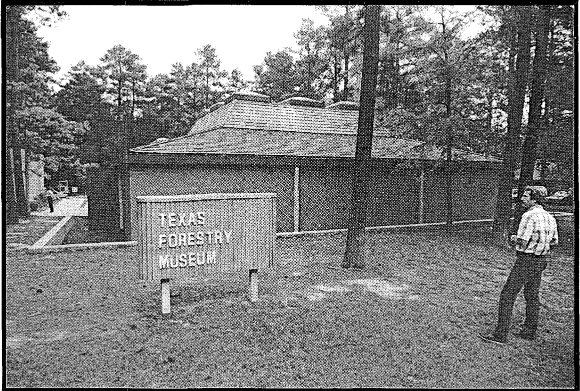
Figure 26. Pressure Treated Southern Pine Roof; 3 Years Old; East Texas
