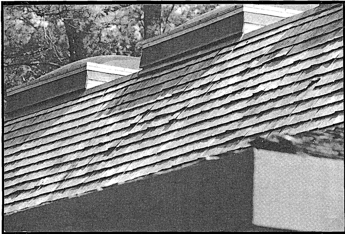
Figure 24. Cedar Roof; 12-15 Years Old; East Texas
