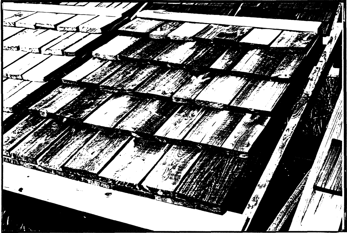
Figure 29. Jack pine - dipped green, Cunapsol. Field exposure test, Hudson, Texas. Installed 7/29/89. Photographed and inspected 2/26/90.
