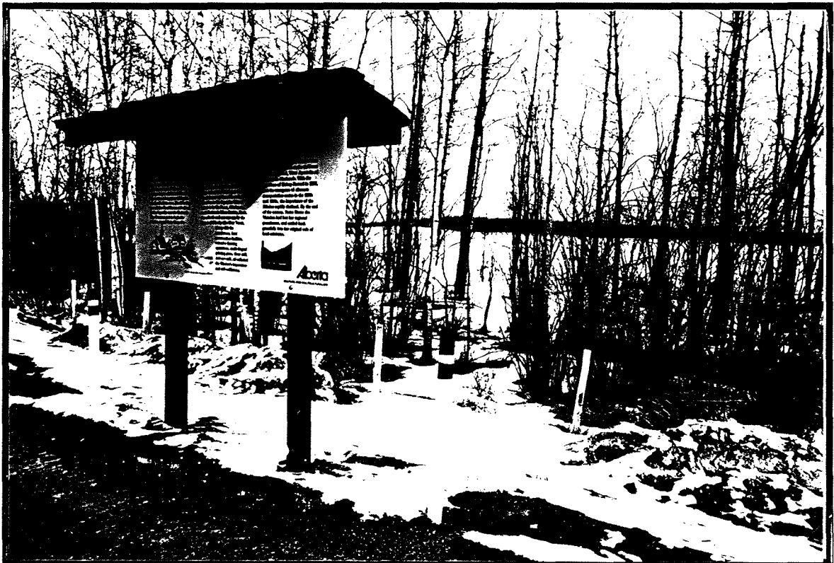
Figure 4. Test roof at Lac La Biche. Jack pine - dipped green, Cunapsol. Installed August 15, 1989.
