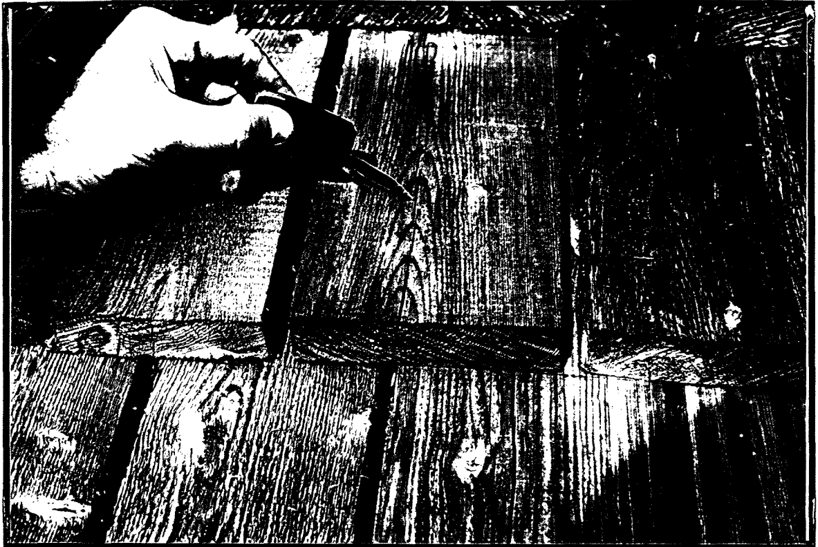
Figure 45. Minor split, flat sawn; Jack pine - untreated; Field exposure test, Hudson, Texas; Installed 7/29/89; Photographed and inspected 2/26/90
