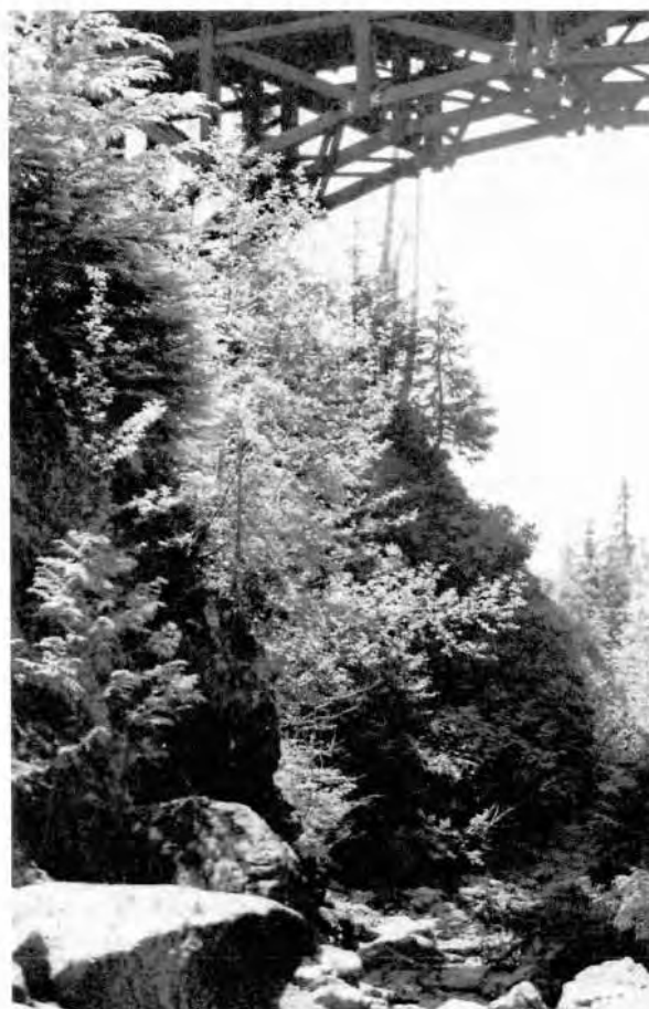
Fig. 32. Many high bridges had to be built along the road to Port Renfrew. The high cost of construction delayed the road for many years.
