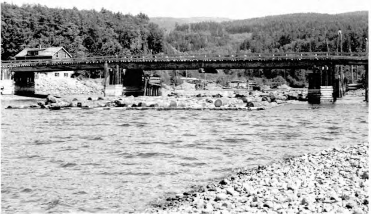
Fig. 15. At Jordan River, logs are sorted, scaled and bundled on dry land. Booms are built in the river mouth and towed away at high tide.
