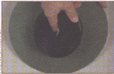
Figure 8 Assembling the lid of the Multi-Pher® trap on the cover of the ABS pipe.
