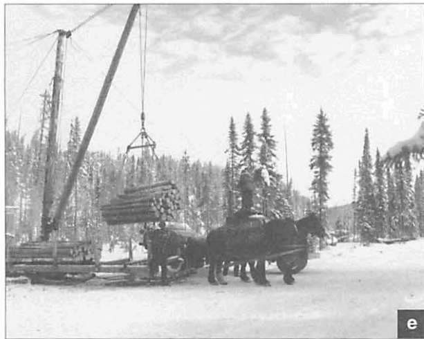
Plate 2. Harvesting in the Black Sturgeon Forest during the 1940s and early 1950s: a. Camp 8 in 1939 (Arnott Whitney); b. Felling with Swede saw; c. Pulpwood piled along skidways; d. Loading pulpwood sleighs by hand; e. Loading pulpwood sleighs with horse-operated jammer winch; f. Skidding and piling sawlogs. Photos 2b to 2f courtesy of Thunder Bay Historical Museum Society, Great Lakes Paper Company collection.
