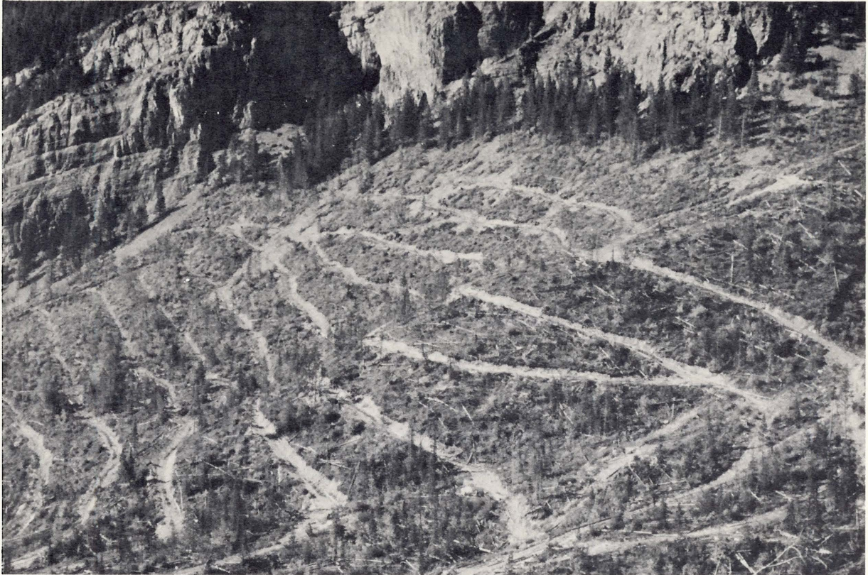
Fig. 1. A ground-skidded clearcut with skidroads built along the contour.
