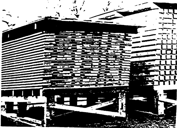
Photo 2 - lumber piled for air drying on a permanent raised foundation
