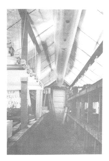
Bench construction using 2"x4" fir and 1"x4" spruce. Both of these benches have been extended to accommodate additional BCFS/CFS trays. Original bench width was 4 feet.
