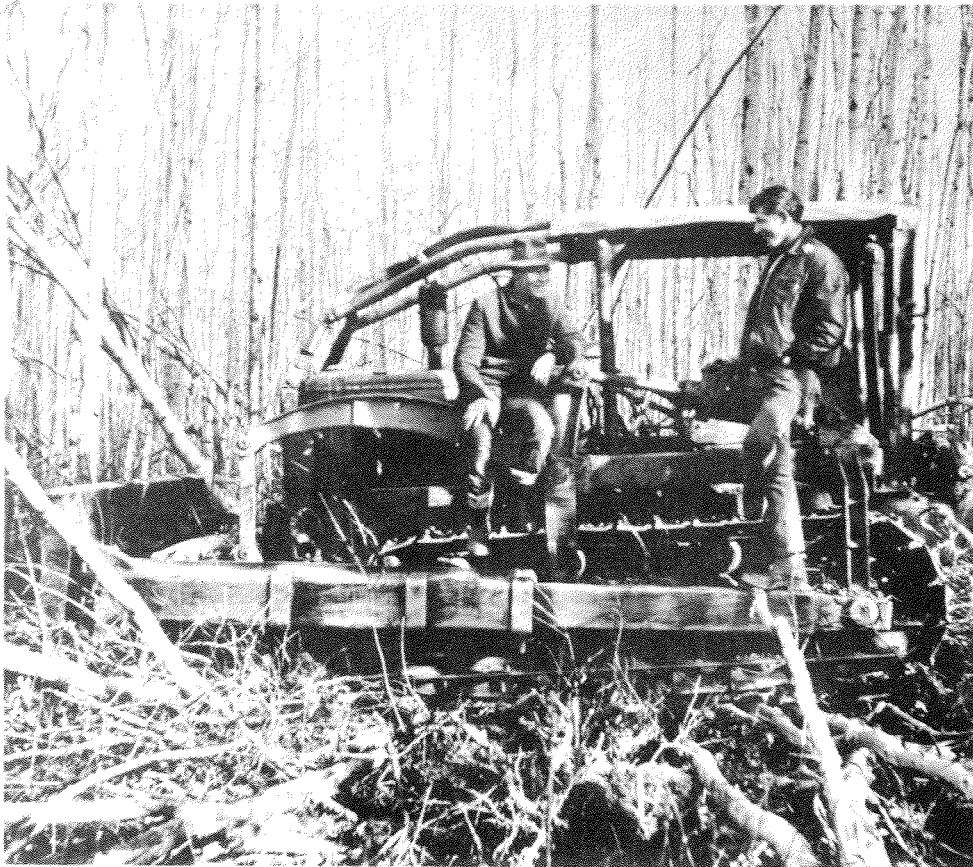
Figure 9. TD-14 Tractor with bulldozer blade.
