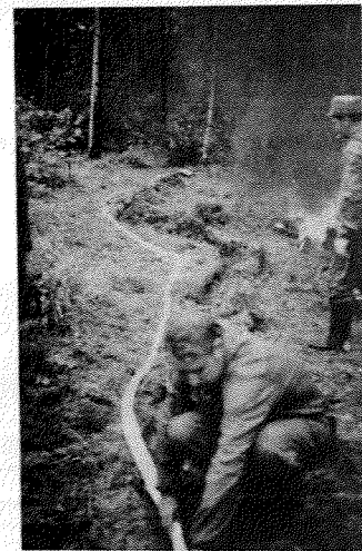
Placing the hose type explosive in a shallow trench (Angarsk)
