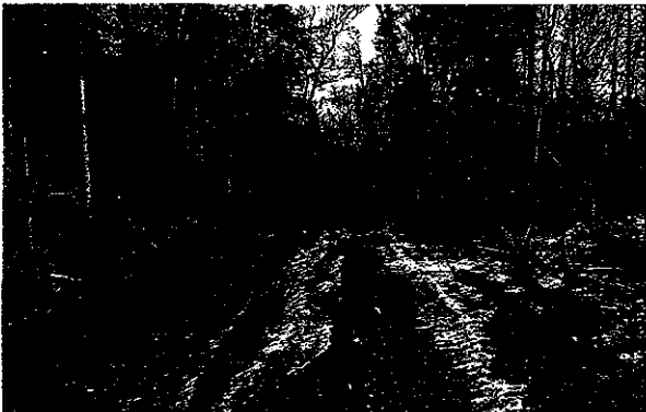
Wood extraction road, large ruts, trucking impossible
