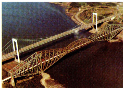
Aerial view of the Pierre-Laporte and Québec bridges.
