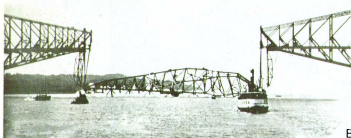
A. The remains of the bridge, August 29, 1907. B. Falling centre truss, September 11, 1916.
