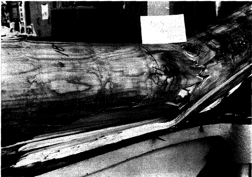
PLATE 6—Typical cup-shaped splintering tension failure.
