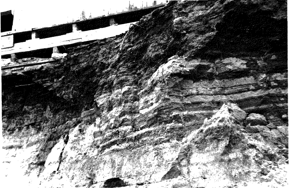
Figure 1. Close-up of the cut bank at Eldorado mill. The land type is alluvial, having stone-free soil containing a moderate amount of buried organic matter.
