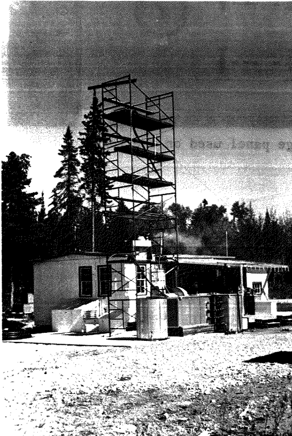
Photo No. 4. Tower for suction lift test.
