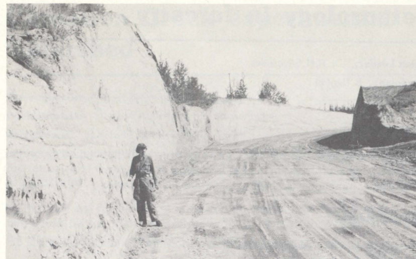
Wind-blown deposit (loess) exposed during highway construction near Teslin Lake, Yukon.
