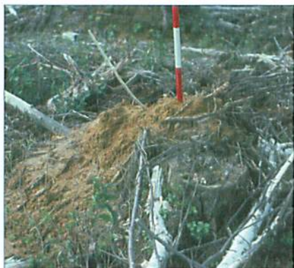
Side berm with logging slash
