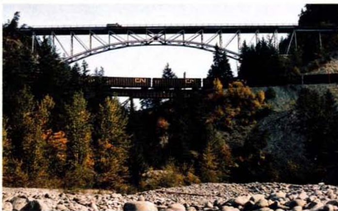
High-level road and rail bridges across Nine Mile Creek
