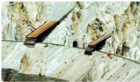
Rock sheds protect the railway line
