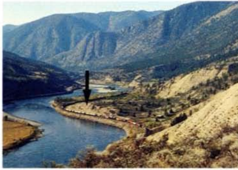
Silt slide that blocked the Thompson River (22)
