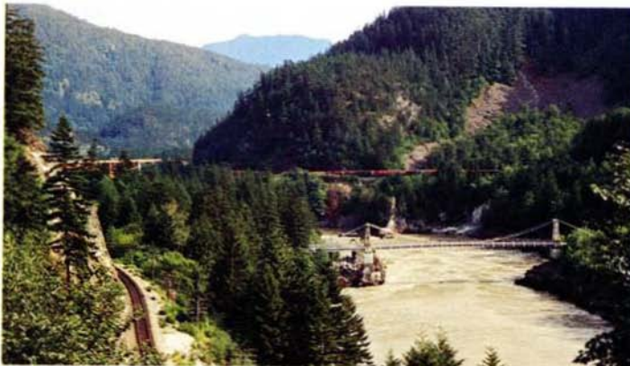
Old Alexandra Bridge in the Fraser Canyon
