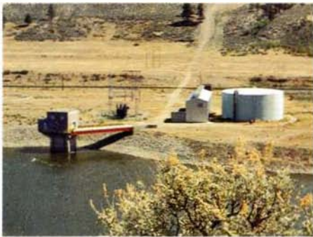
Water pumping station
