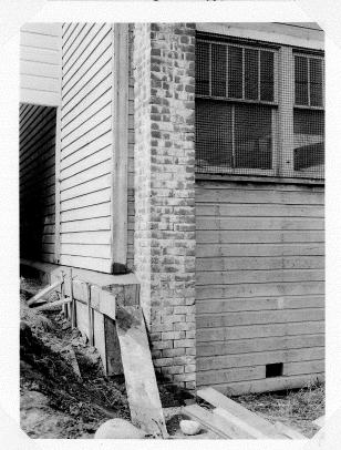
Same building as above, showing concrete replacement work undertaken as result of termite attack. Vancouver, B.C.
