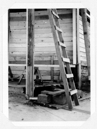
Front of store being rebuilt as the result of termite and rot damage to foundation timbers. Vancouver, B.C.
