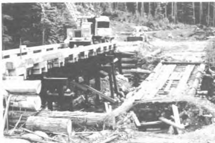
Figure 3 A Glu-Lam bridge replaced the old log stringer bridge across Wilson Creek near Mile 7½.
