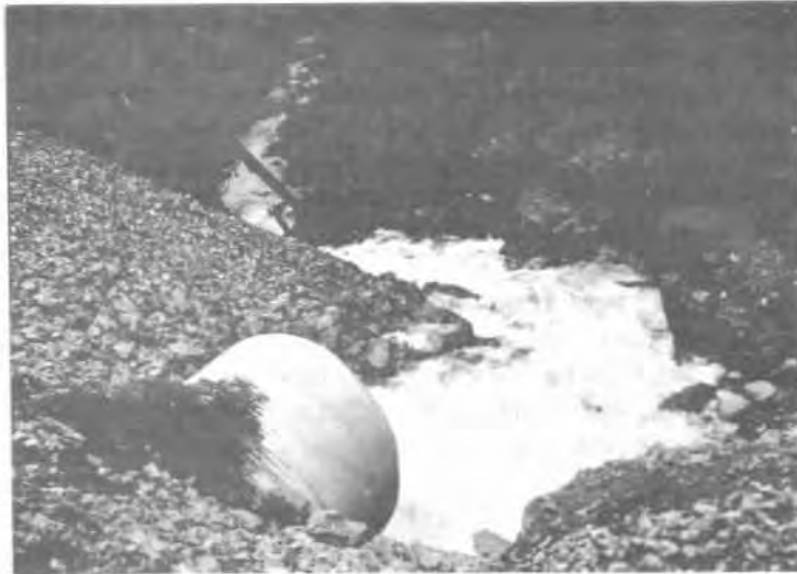
Figure 4 Outlet of the culvert at Hicks Creek.
