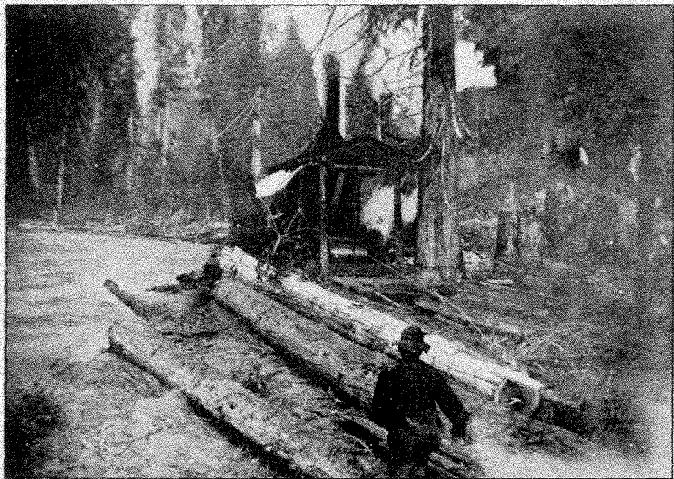
In the Lumber Woods at Fish River, B.C., showing Donkey Engine used in drawing out Logs.
