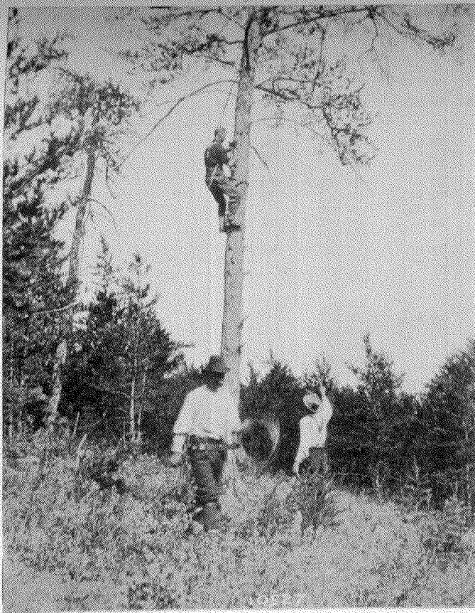
Forest protective equipment. Forest rangers constructing a tree-line telephone system, Nisbet forest reserve, Saskatchewan
