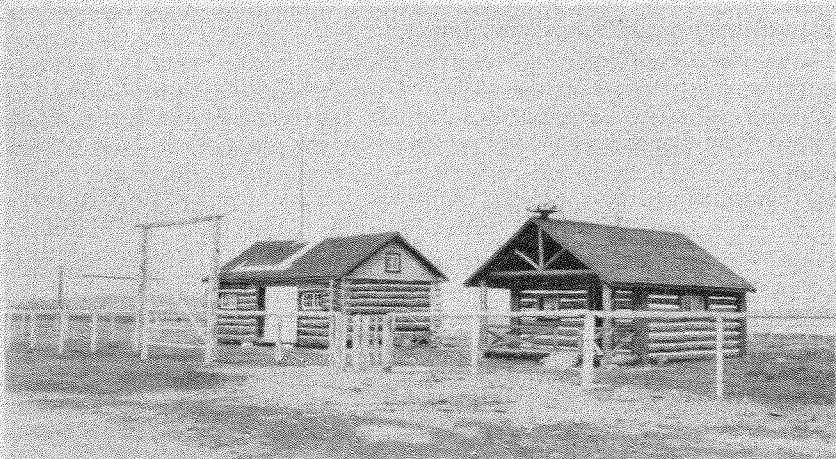
PLATE NO. 8.—RANGER CABIN AND WAREHOUSE AT ILE À LA CROSSE, SASKATCHEWAN. (F. S. Photo. 19848)
