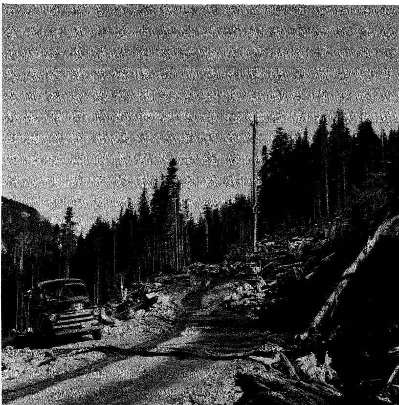
FIGURE 3—A 90-foot portable steel spar.
