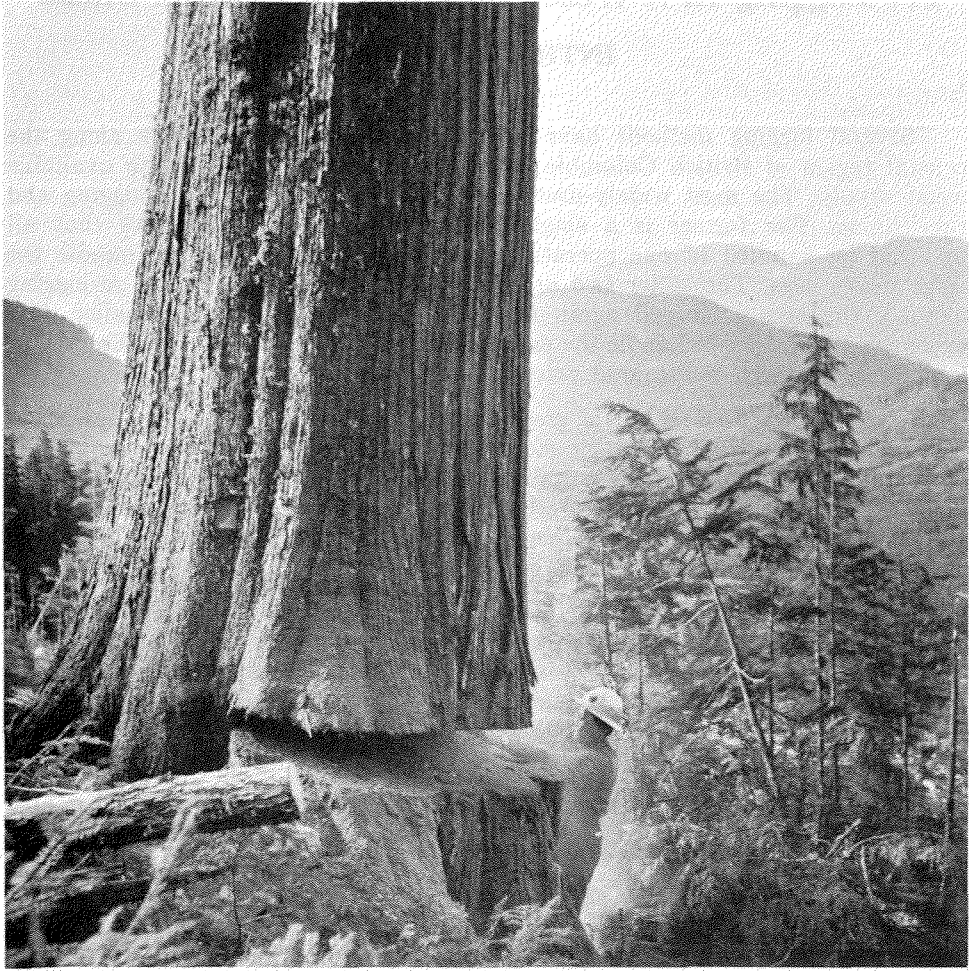
FRONTISPIECE—A "Humbolt" undercut in a large cedar—note the angle of the cut and also the low stump.
