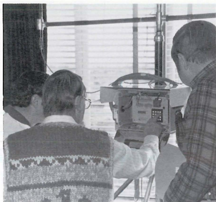
Staff are shown here examining a typical installation.
