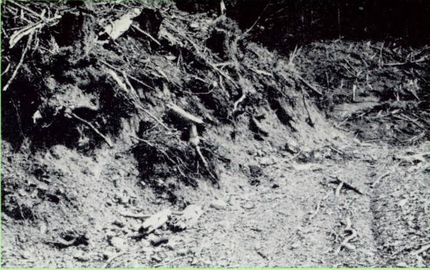
Skidroad constructed on a steep slope.
