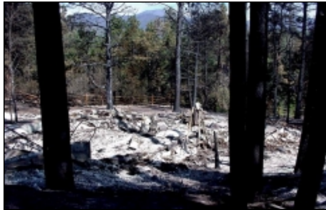
Photo 4—The unconsumed, moderately scorched tree canopy along with the remaining wood rail fence indicate that this home was exposed to a low intensity surface fire. The high intensity wildfire burned on the hills in the background.
