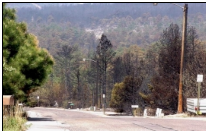
Photo 10—This is a portion of the area within the yellow rectangle shown in the previous photo. The trees burned from the burning homes. The homes ignited from the low intensity surface fire and adjacent burning homes.
