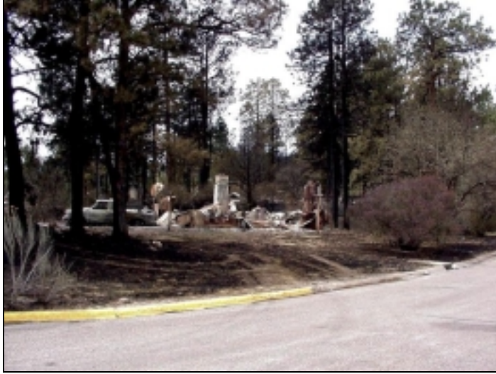
Photo 5—This totally destroyed home was within the residential area. A road separated it from other burning vegetation and homes. The unconsumed vegetation with little scorch indicates that the fire intensity surrounding the home was low. This suggests that firebrands (burning embers from other fires) ignited the home directly and/or in adjacent flammable materials that spread to the home.
