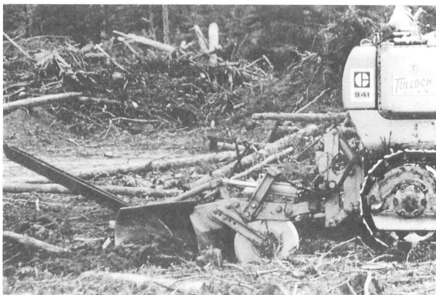
Figure 6. The Michigan floating parallelogram hitch attaches the fire plow to the bulldozer for use as a scarifying tool in this instance.
