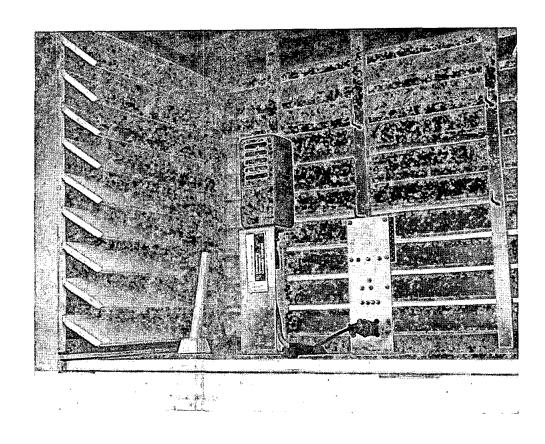
Photograph No. 2. Relative humidity (left) and air temperature (right) sensors of the Remote Control Fire Weather Station in a Stevenson Screen at field location. July, 1968.
