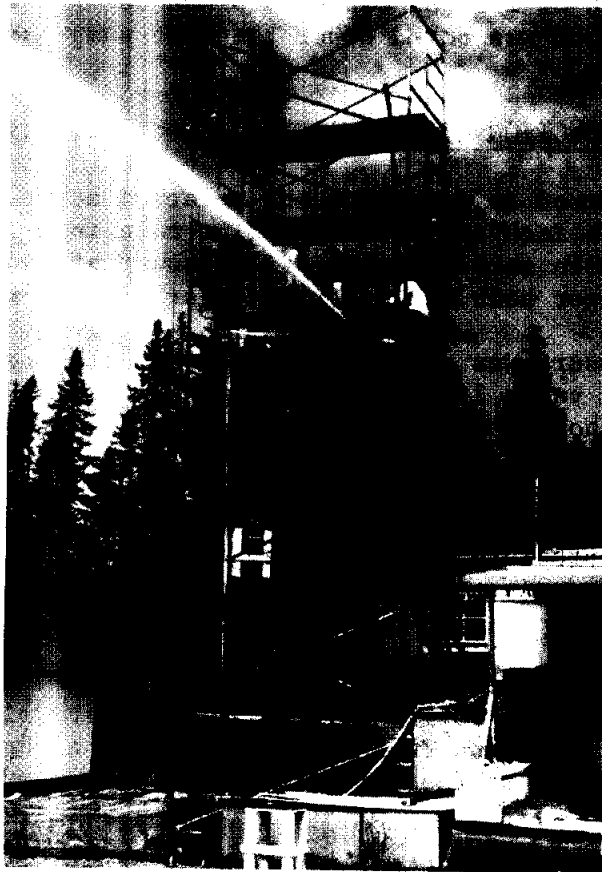
Photo No. 8 Tower for suction lift test.
