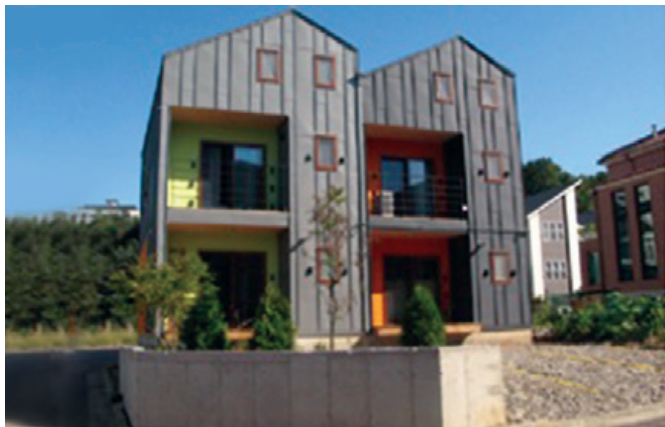
Korean semi-detached house. Photo courtesy of Hyun Wook Lee, architect
