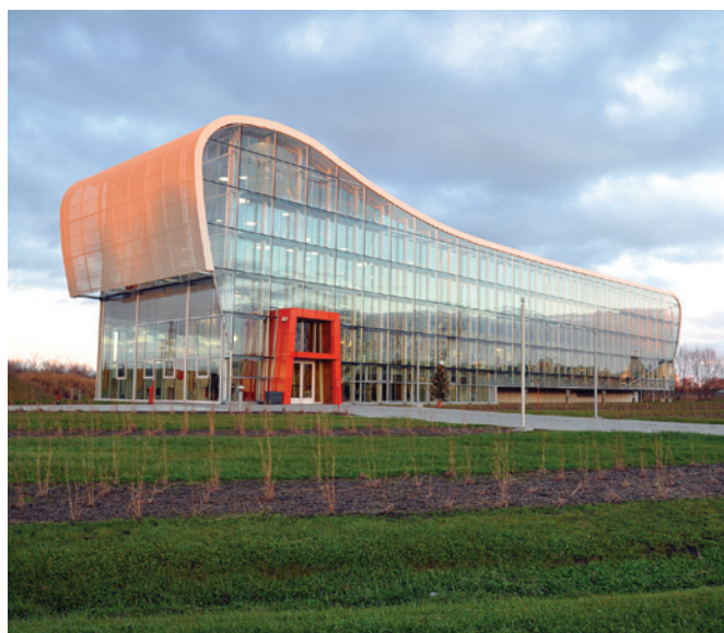
GlaxoSmithKline Administration Building. Photo courtesy of FPInnovations
