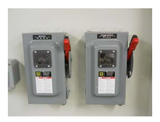
1.4.3 The Groen cooker/mixer is powered from two sources. Ensure that power is disconnected at both the wall receptacle and the circuit breaker before assembling, disassembling, servicing or cleaning.
