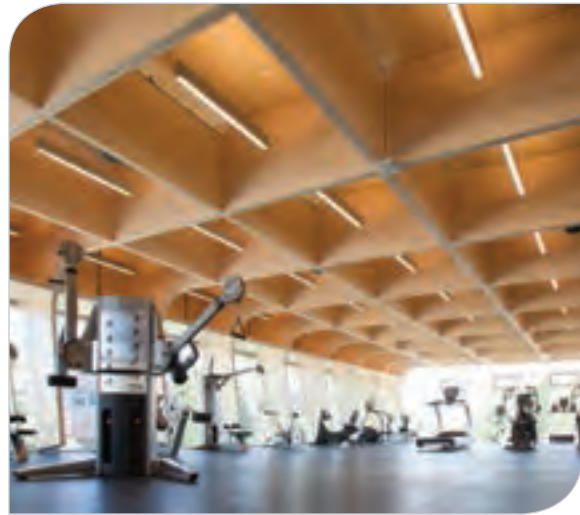
The new multi-use wellness building at the University of British Columbia Okanagan Campus was the first to be constructed using cross-laminated timber for beams. Photo courtesy of Structurlam Products LP.
