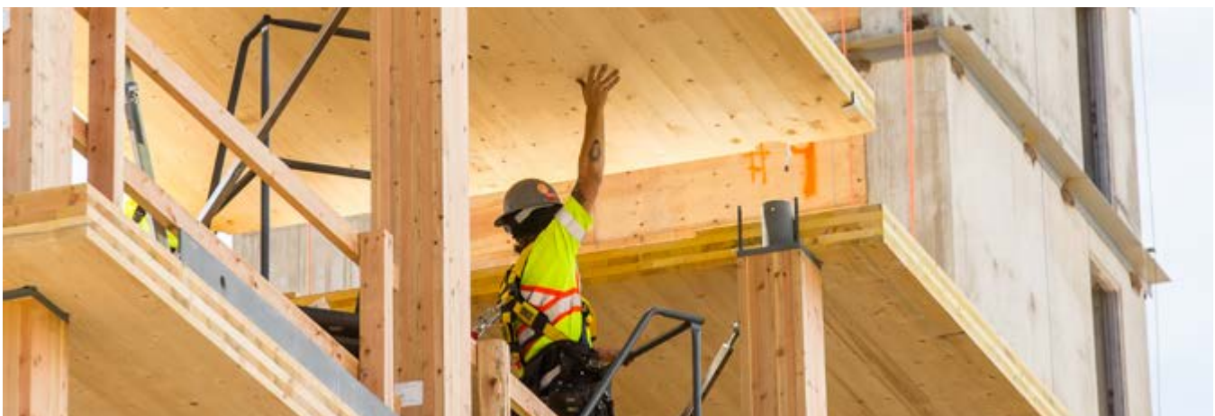
Advanced materials made from wood are used in the construction of mid-rise and tall buildings – 6, 10 and even 18 storeys high.
