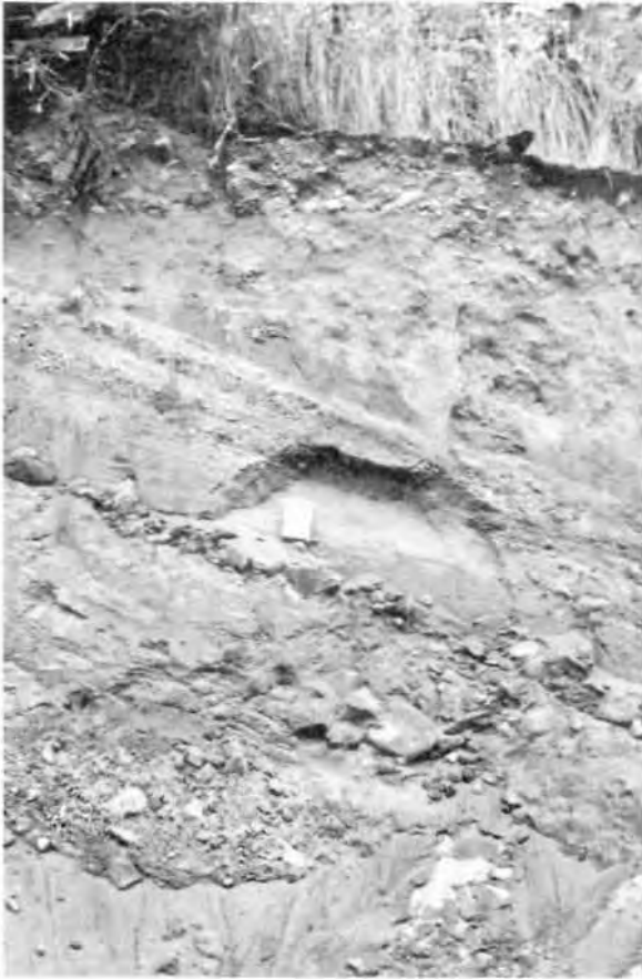
FIGURE 25 - A deep deposit of alluvium. Note the tilted layers deposited while the island was depressed and the overlying layer of outwash material. This is a source of borrow material for construction purposes.
