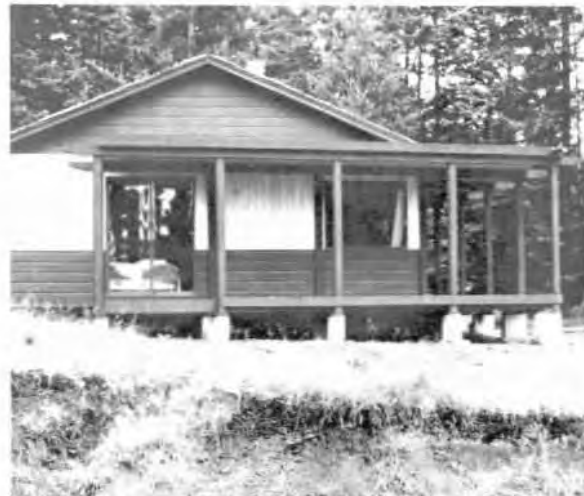
FIGURE 22 - A house built on cement supports to allow drainage.
