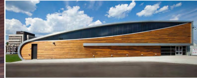
The UQAC Arena features a hybrid wood-steel truss system supporting a glulam deck.
