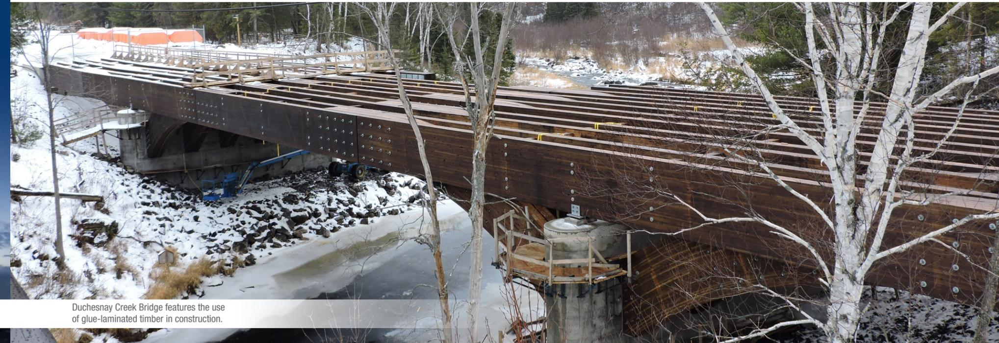
Duchesnay Creek Bridge features the use of glue-laminated timber in construction.
