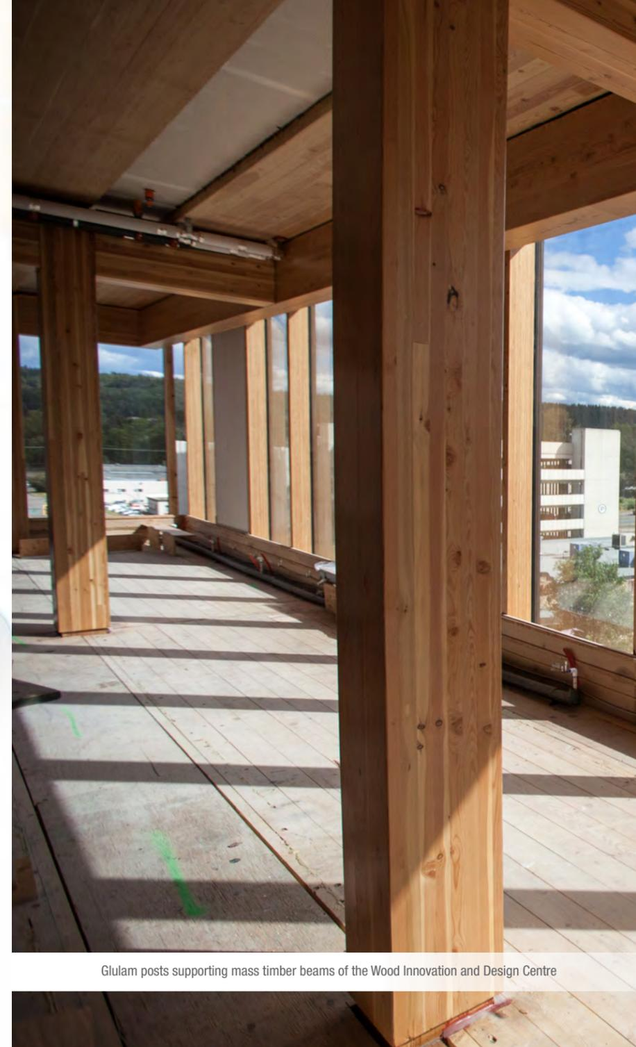
Glulam posts supporting mass timber beams of the Wood Innovation and Design Centre
