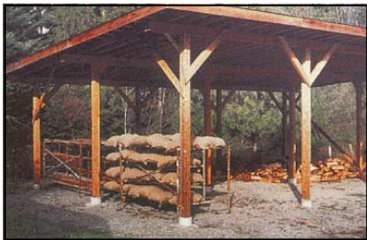
FIGURE 23. Interim storage of Douglas-fir cones
