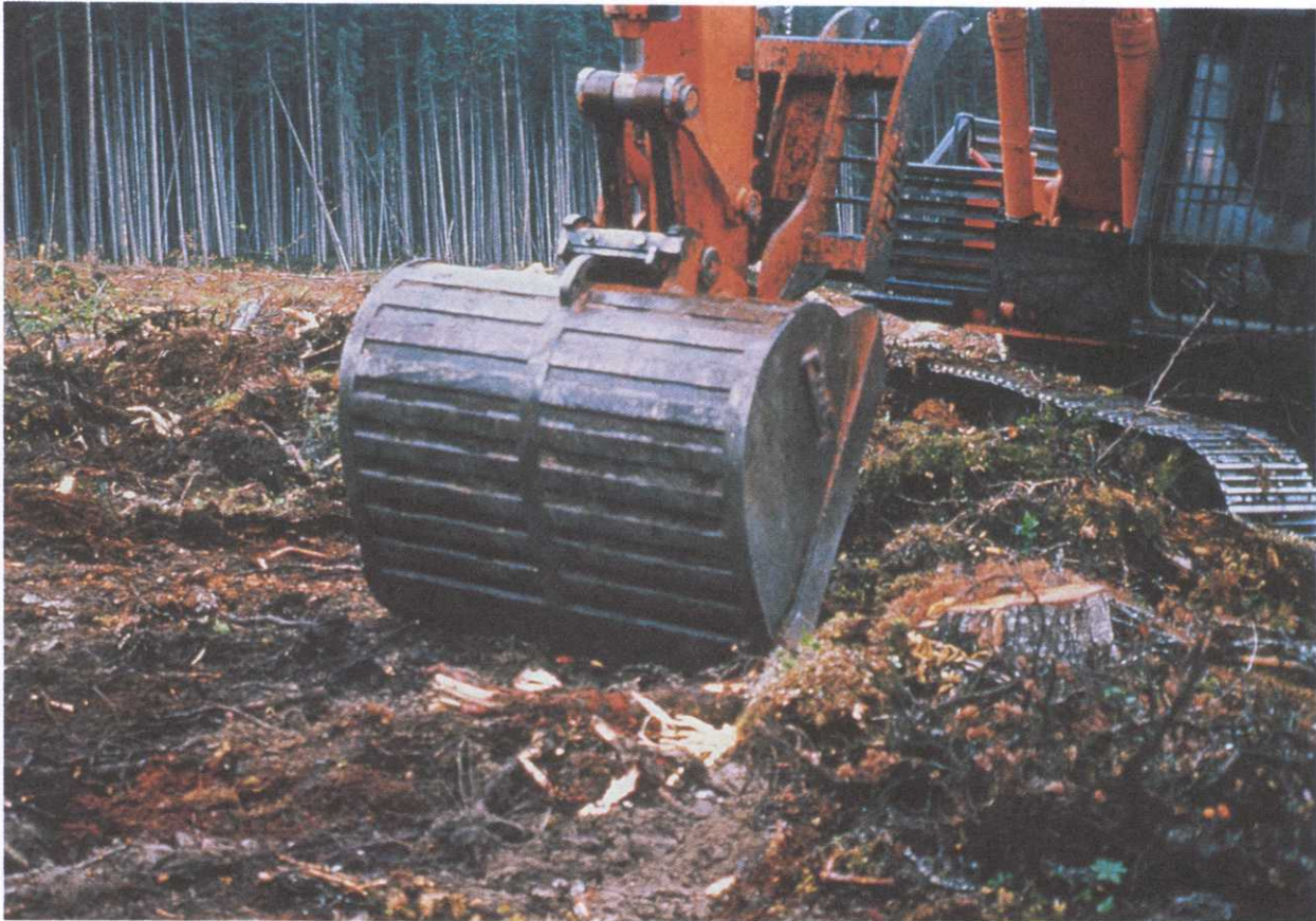
FIGURE 6. Bucket on backhoe was used to peel off the forest floor.
