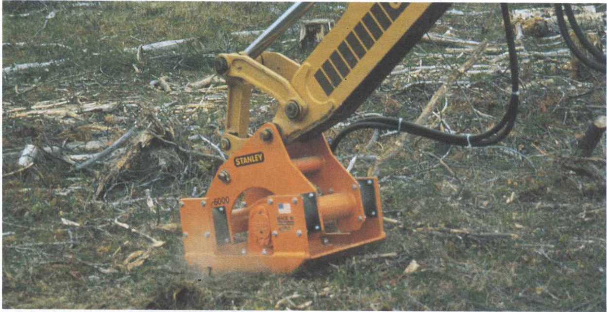
FIGURE 7. Tamping plate on backhoe was used to compact the mineral soil.
