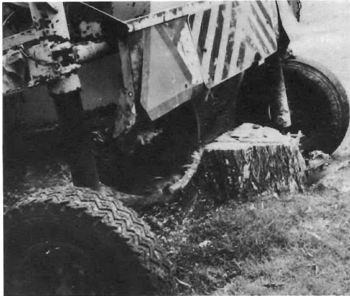
Removing a stump using the stump grinder
