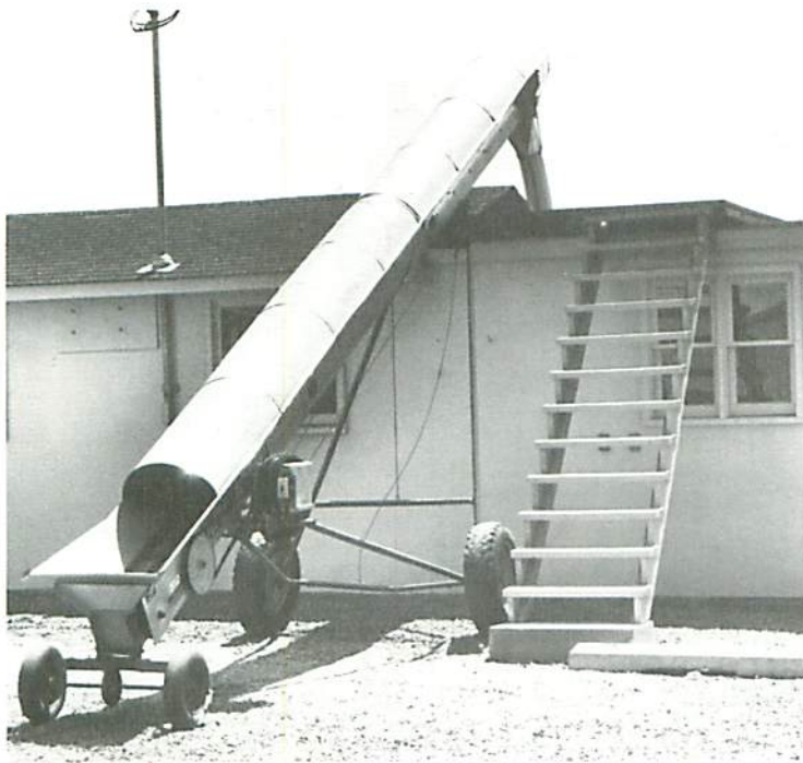
Fig. 9. Header-house and peat conveyor.
