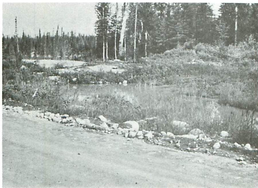
Figure 6. Small depression acts as a sediment pool.
