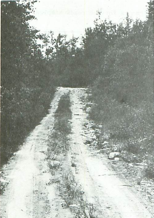
Surface erosion and deposition
