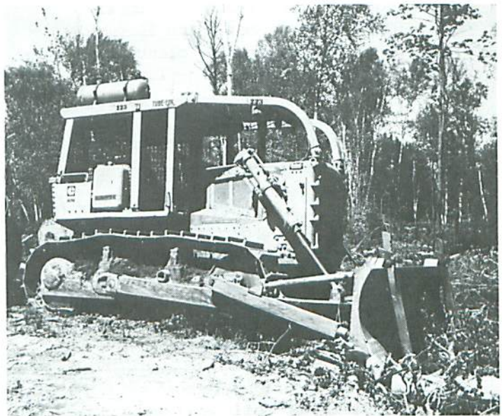
Figure 4. Two Young's Teeth mounted on Caterpillar D7G bulldozer
