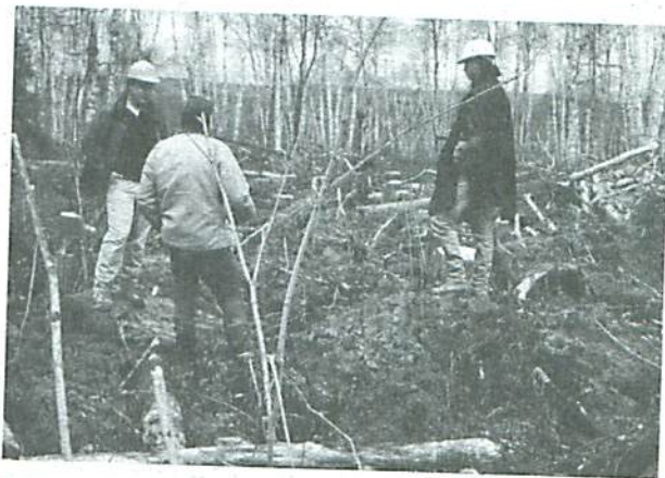
Figure 4043.1. Inspecting the mounding site treatment following preparation, but prior to planting. (Photo courtesy of Dr. R. Sutton.)
